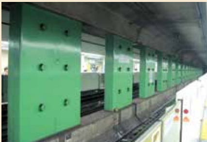
Reinforcement of the central pillars of the platform
